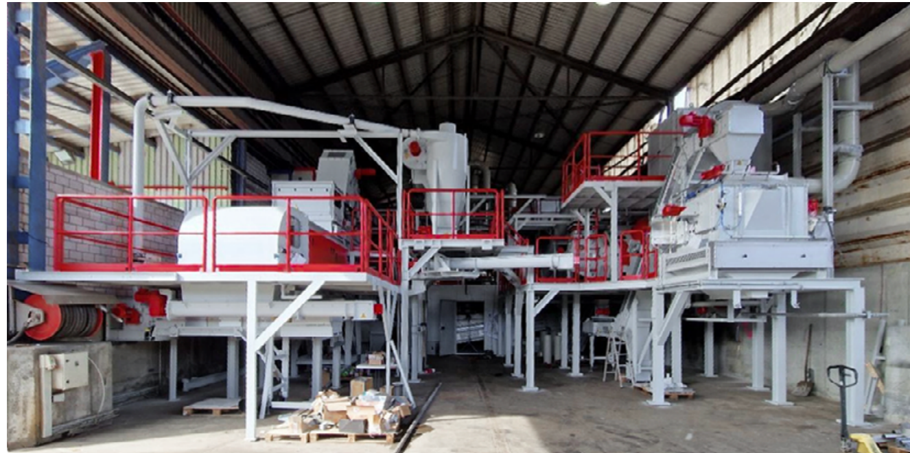
E. Flückiger AG refrigerator recycling plant from URT under construction. Left: eddy current separator, right: pellet cooler.
